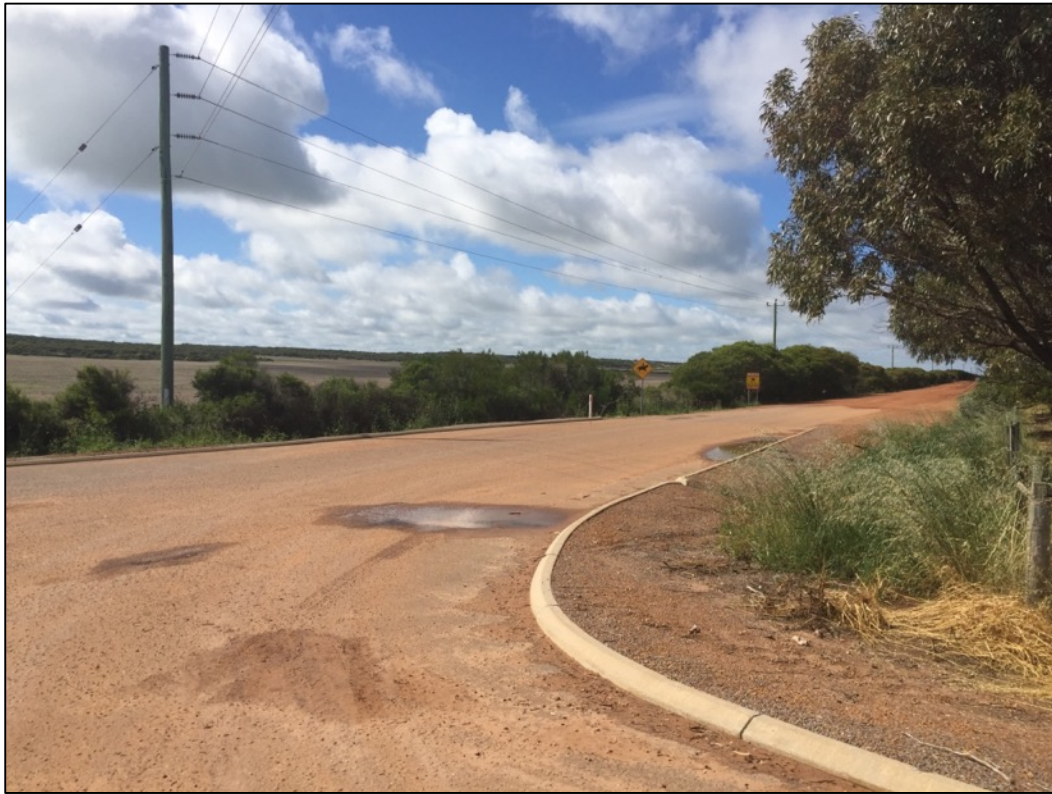
Figure 9 – View of fishtail from Hampton Road onto Jandalool Road
